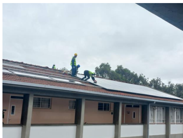
Good progress on Imani House
